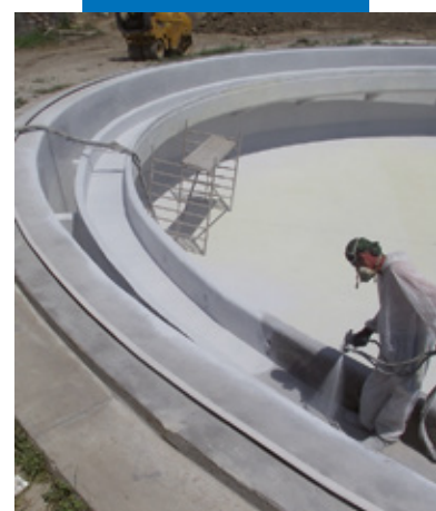
Application of Purtop 1000 onto industrial storage tanks
