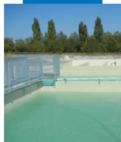
Storage tanks waterproofed with Purtop 1000
